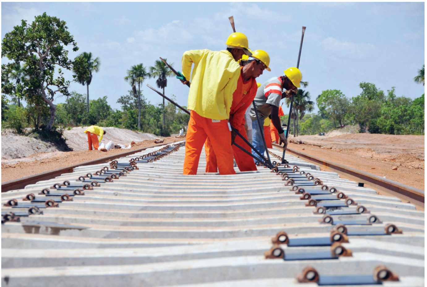
Tracklaying underway on a section of the North South Railway.
